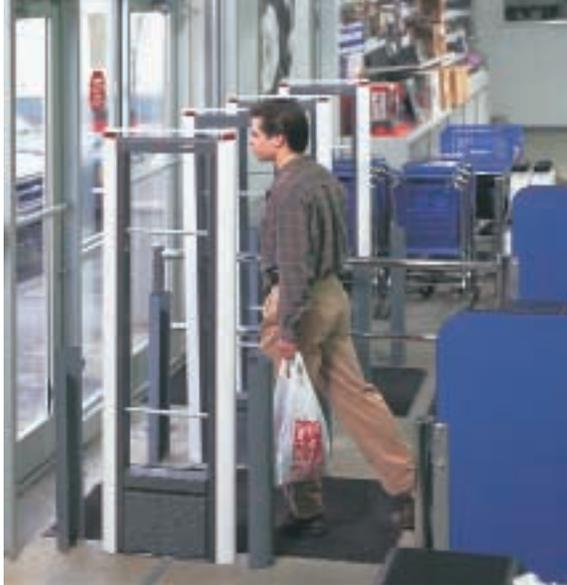
envelope of RF energy, RF sensors recognize RF tags or labels passing through which results in an alarm. And, all RF sensors detect embedded, source tagged RF labels that have not been deactivated at checkout.
